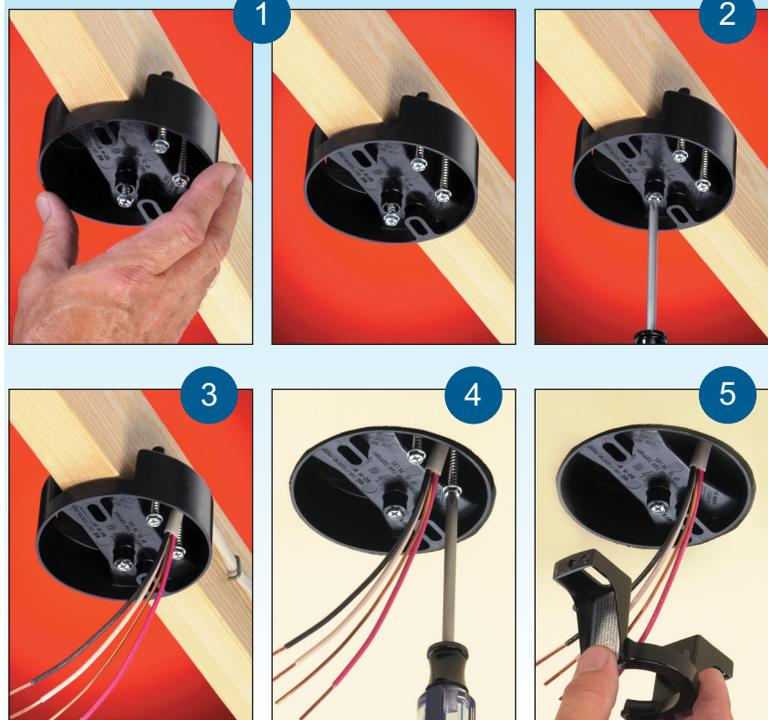
1. Press box onto joist. Gripping tangs hold the box in place temporarily.
