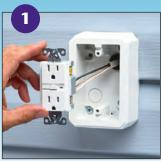
Remove KO from FS Box and insert NM cable connector. Push cable through connector and position box onto siding.
