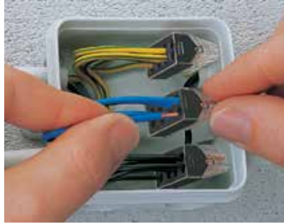
Then insert stripped conductor firmly into connector. Check for complete insertion through clear/transparent housing.
