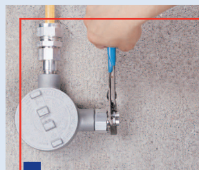
5 Insert adaptor on enclosure.
