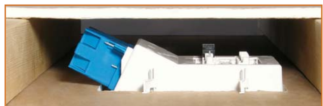
Top view showing ample room between drywall and studs
