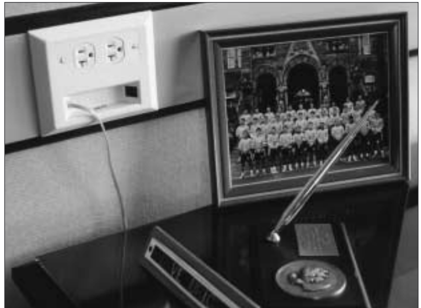
Access 5000 Raceway installed at chair rail height.
