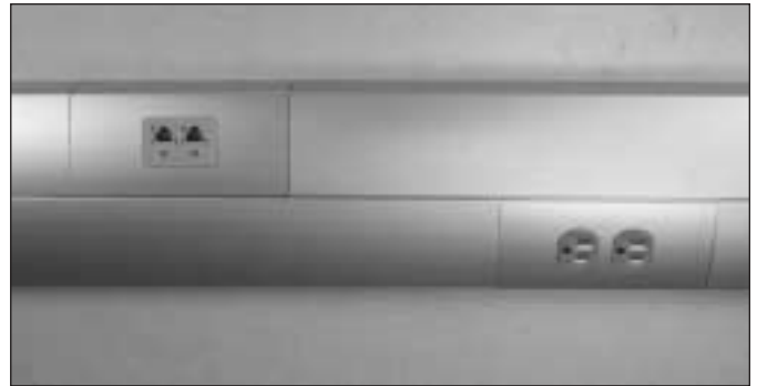
ALDS4000 Series Raceway installed with front data and power activations.
