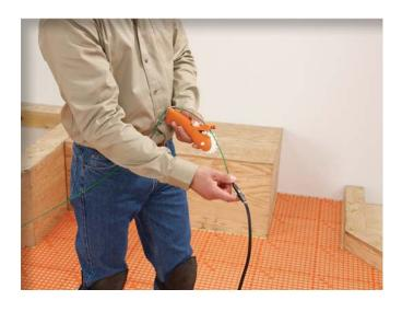
The FLEXGlide's wheel is perfectly matched with the FLEXSnap mesh to ensure an easy and uniform installation of the heating cable, even when changing directions or going around obstacles..
