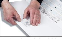
Step 5: Insert the sensor back into the hole. The sensor may or may not require a socket.
