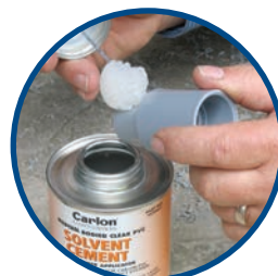
Apply a uniform coat of cement.
