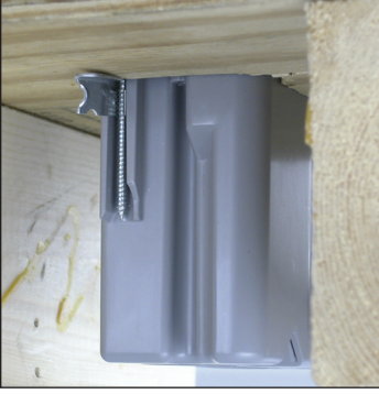
Integral swing tabs hold box securely to the floor from below.
