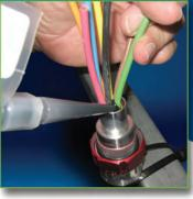
Finally, fill the sealing chamber while manipulating the de-energized conductors to encourage sealant flow.
