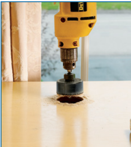
Included hole saw attaches to a power drill for quick and easy installation.
