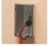
Completed installation with weatherproof-in-use cover. DBVM1C shown.
