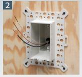
Install NM cable connector and wire. Attach recessed IN BOX to substrate, then install moisture barrier around box as shown above in Method 1.
