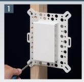
Install NM cable connector and wire. Attach IN BOX to stud.
