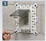
Install NM cable connector and wire. Attach recessed IN BOX to block. Holes in flange allow stucco to bond firmly.
