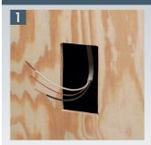
Make a 3-1/4" x 5-1/2" hole in plywood. Pull wiring through opening.
