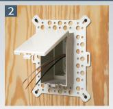
Install NM cable connector and wire. Attach recessed IN BOX to plywood.
