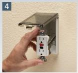
Install wiring device per manufacturer's instructions, Local, and National Electrical Codes. Accepts most devices and a standard indoor wall plate.
