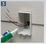
Cut rigid siding to fit around IN BOX. Caulk around box.
