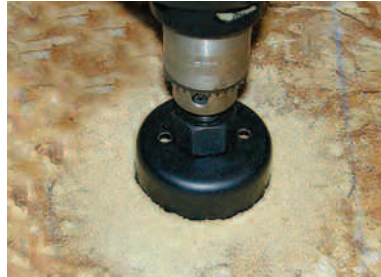
2. Drill hole in floor using hole saw.
