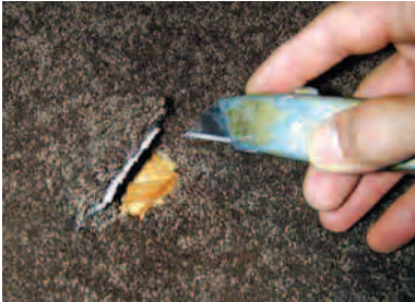
1. Cut 2-3/8" hole through carpeting before using hole saw.
