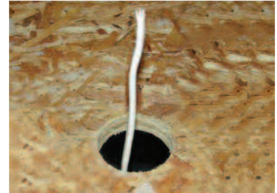
3. Pull cable through floor.
