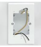
STEP 4 Wrap bare ground wire under ground screw head on recessed metal ground strip - Part #3 and tighten down. Install siding or stucco or masonry around box and add drip edge and/or caulking as needed.
