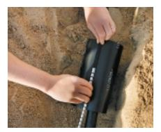
Sleeve is positioned over splice or damaged area and closed with metal channel.
