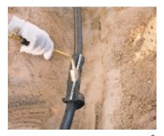
Heat is applied to shrink the sleeve and melt the adhesive liner.
