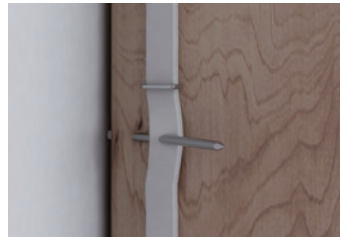
Inadvertent nails can puncture wire behind wall
