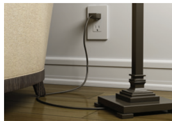
Electrical cords can be damaged under or behind furniture
