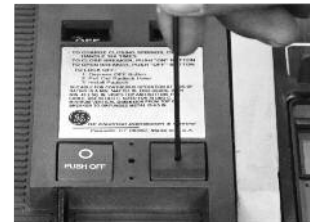
Activating the switch closing mechanism through the hole in the Hidden "ON" Button
