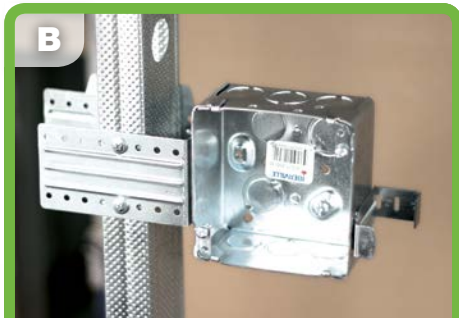
B When box supported on stud, align box and attach bracket firmly with steel screws to front and rear.
