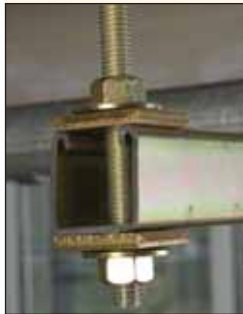
Standard method using nuts and washers
