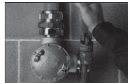
5. Install hub on enclosure
