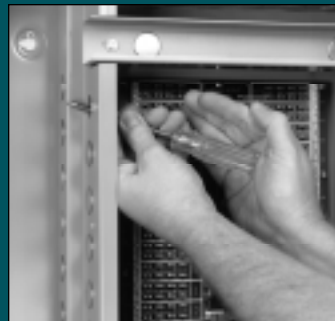
5. Remove knockout plugs from panel.
