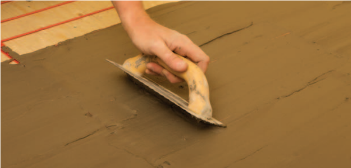
FIGURE 2.52: Thinset mortar method
