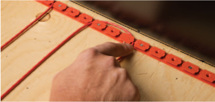
FIGURE 2.26: Install the heating cable
