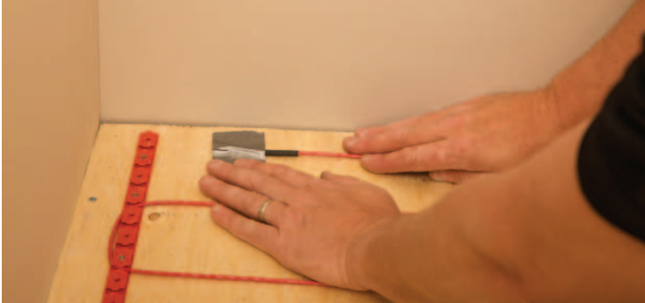
FIGURE 2.28: Secure the end seal
