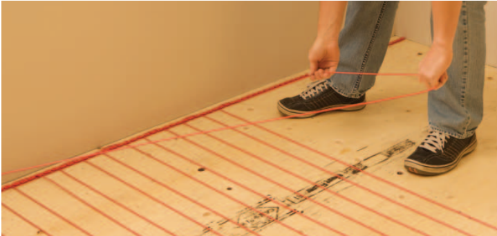
FIGURE 2.27: Install the heating cable
