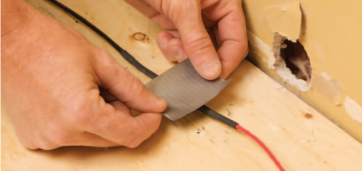
FIGURE 2.23: Secure the cold lead to the subfloor
