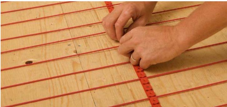
FIGURE 2.29: Install stabilizing guides
