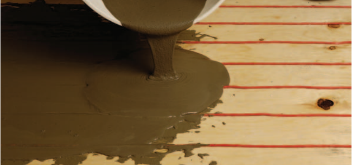
FIGURE 2.42: Self-leveling compound method
