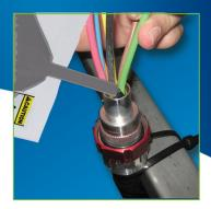
Finally, fill the sealing chamber while manipulating the de-energized conductors to encourage sealant flow.
