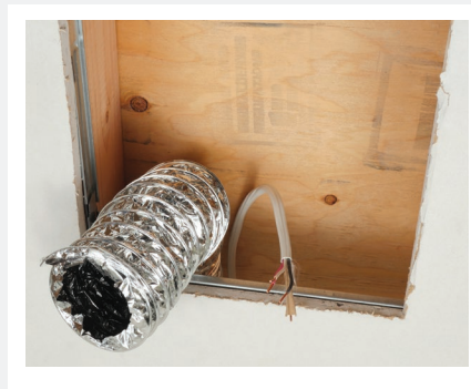
Existing 3" Duct and wiring
