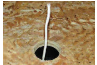
3. Pull cable through floor.
