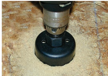
2. Drill hole in floor using hole saw.
