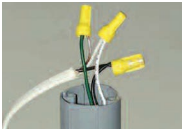
4. Connect receptacle wires to cable. Be sure to match wire colour(s).
