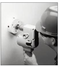
Determine location and cut hole in wall using a hole saw, keyhole saw or a core drill.
