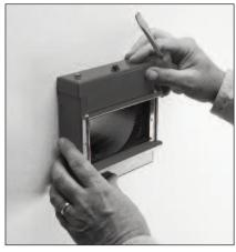
3. Place the FlameStopper Thru-wall Fitting Box over the opening and secure the two bolts.
