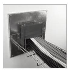
5. Attach FlameStopper box to split conduit.
