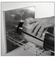
2. Attach ceramic heat protected wall plate to cover irregular hole cut. Insert split conduit around existing cables.
