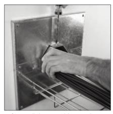
Screw wall plate to conduit to complete assembly.
