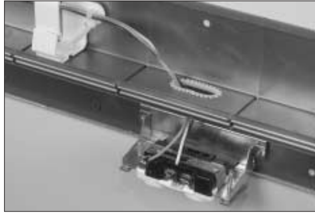
Mount Bracket in lower channel with Screws removed.
