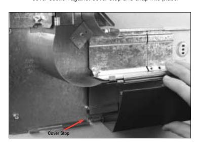
**Step 5.** All Fitting Covers snap into place. Tabs on Fitting Covers align with slots in Fitting Base.
