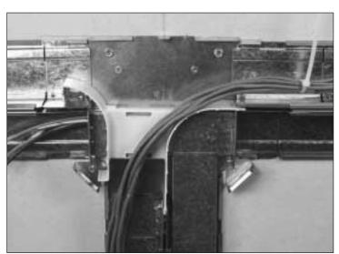
**COVER INSTALLATION:** Hook corners as shown and snap into place.
