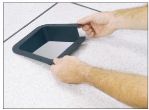
5. Place outer ring (A) and fabric (B) grommet over gasket (F), and secure outer ring<sup>‡</sup> (A) to raised floor using the self-tapping screws that are provided. This ensures a pathway to ground to prevent buildup of electrostatic charge. Note: A 3/32" pilot hole is recommended for concrete filled panels.
