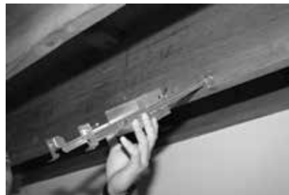
Step 2: Use the rotating hanger bar clip to pivot the unit into position
