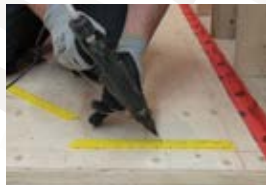
UNIVERSAL GAUGE INSTALLATION (included)
