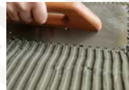
THINSET MORTAR APPLICATION
