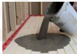
SELF LEVELLING MORTAR APPLICATION
