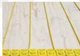
HEATING CABLE INSTALLATION
