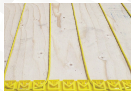
HEATING CABLE INSTALLATION
