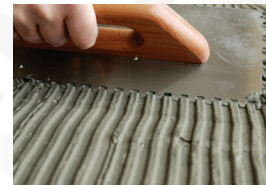
THINSET MORTAR APPLICATION
