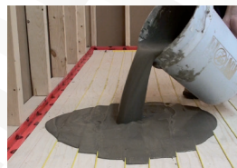
SELF LEVELLING MORTAR APPLICATION
