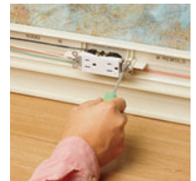
Wire and mount devices in the raceway.
