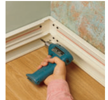
Screw base sections into mounting elbows and wall.
