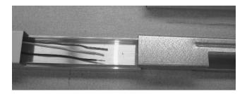
5. Tighten coupling hold-down screw.
