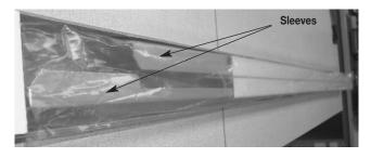
2. Remove the 8" [203mm] cover from the top of 25DTP-4 Tele-Power Pole.
