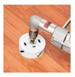
1 With a hole saw cut a 5" diameter hole through flooring and subfloor.
