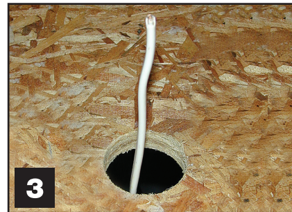
Figure 3 - Pull NM Cable through floor.
