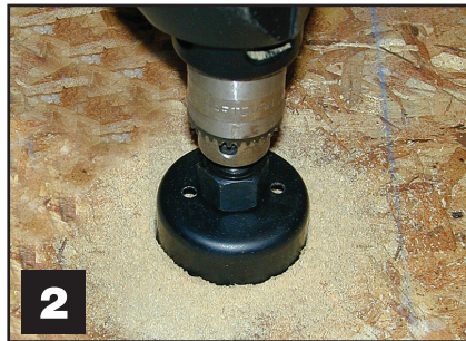
Figure 2 - Drill hole in floor using a hole saw.
