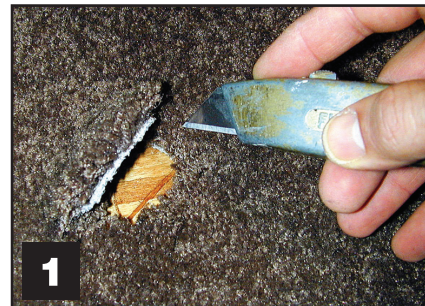
Figure 1 - Cut 2-3/8" hole through carpeting before using a hole saw.
