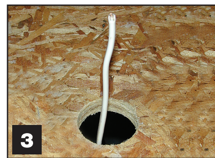
Figure 3 - Pull NM Cable through floor.
