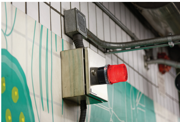
Single and Multicolor Warning Light is used for long distance signaling
