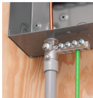
PVC pipe works with GB5T
