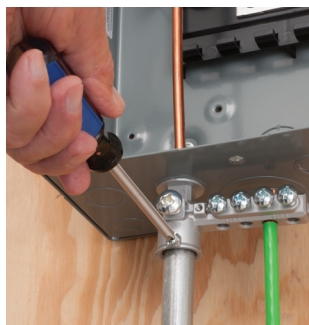
Installing EMT using set screw
