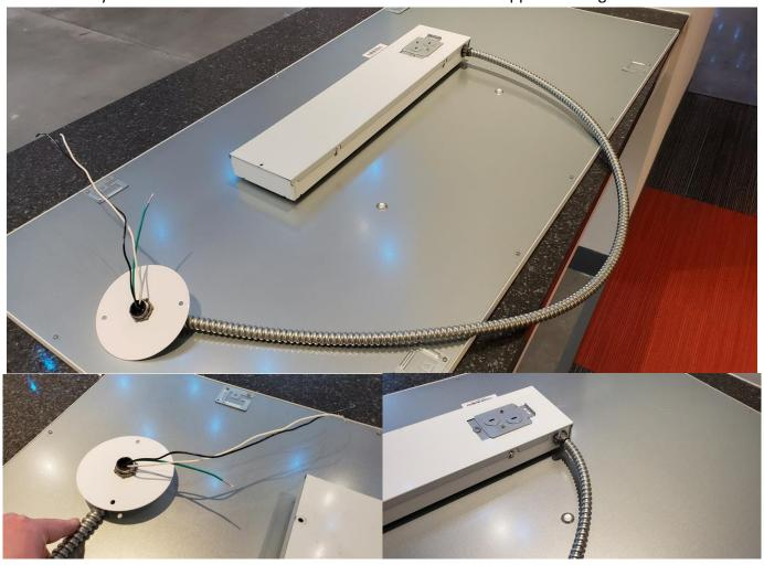
4. Slide fixture into surface mount and make final connections from whip/j-box cover to j-box.
