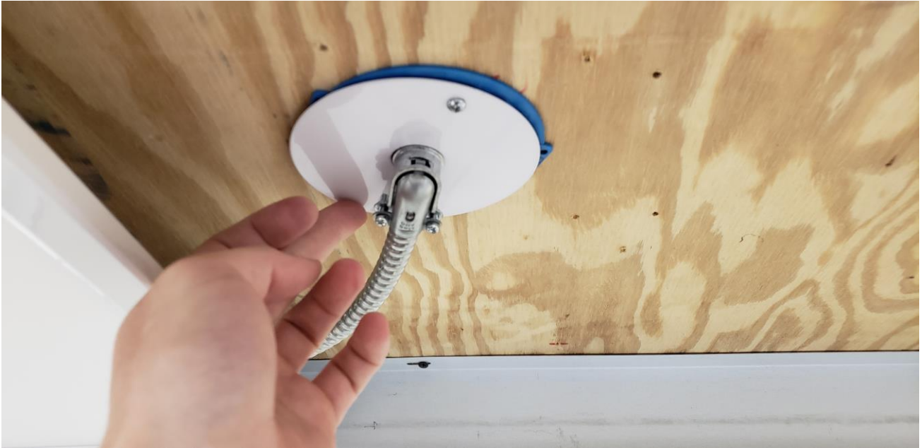
5. Push fixture all the way in and fasten the remaining end cap.
