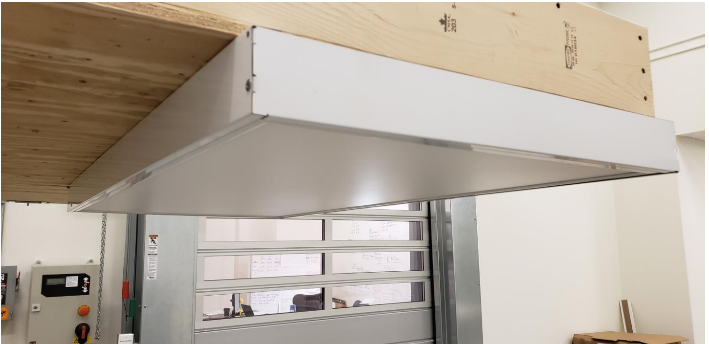
5. Push fixture all the way in and fasten the remaining end cap.
