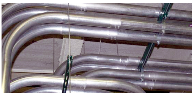
Faster EMT Installations
