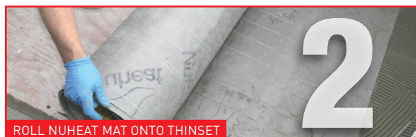
ROLL NUHEAT MAT ONTO THINSET
